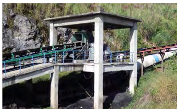
Start point of the coal conveyor to the power station
