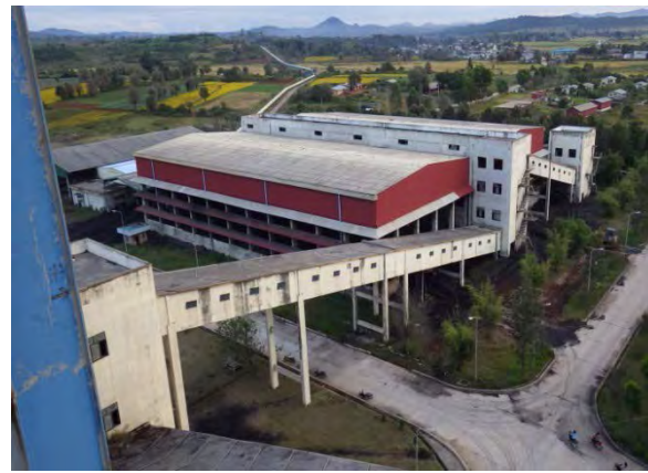
(from the depth) Conveyor from Coal Mine, Indoor Type Coal Storage Yard, Conveyor to Boiler Bunker
