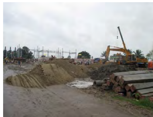
240MW GT Construction Site
