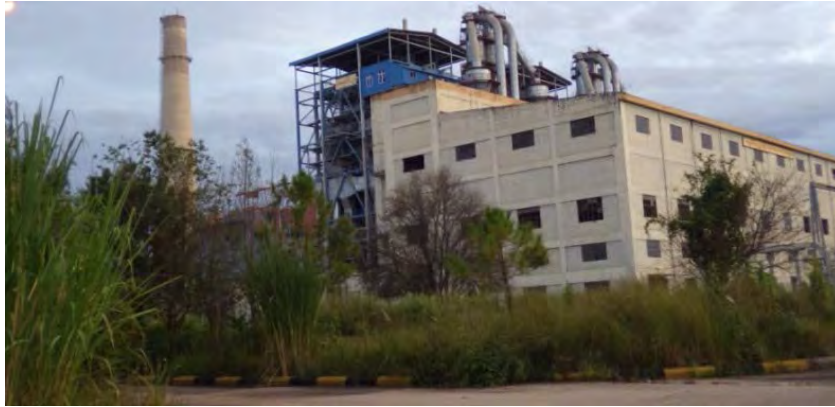
(from right to left) Turbine House, Boiler, Stack
