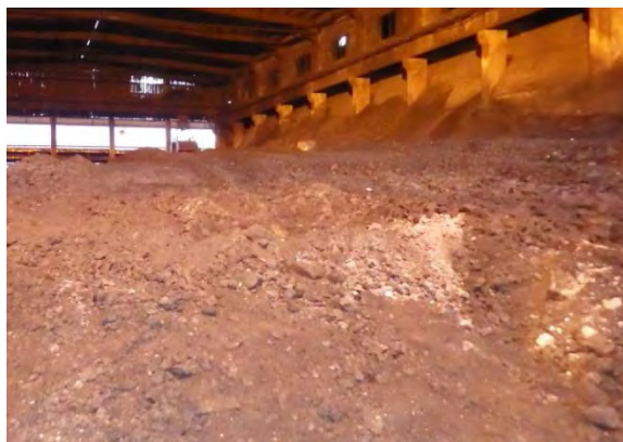
Indoor Type Coal Storage Yard
