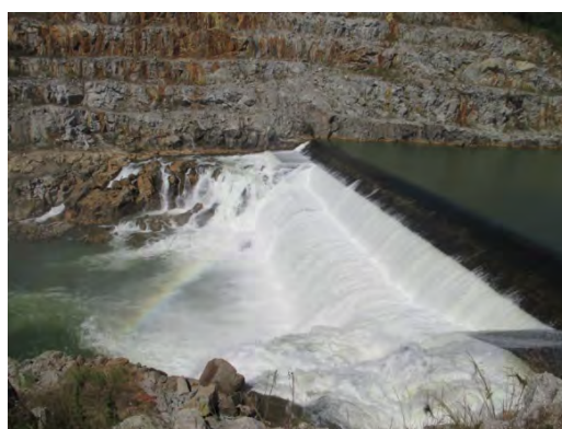
Spill out from spillway
