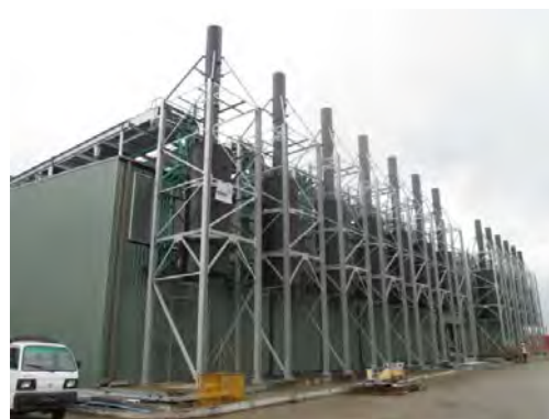
52MW GE Plant
