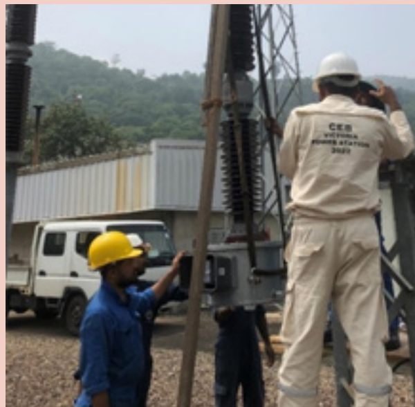
Figure G3: CVT installation in progress
