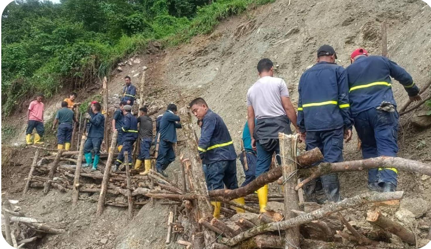
Protection of the tower against landslides, along with the simultaneous installation of an ERS tower for worst-case scenarios.
