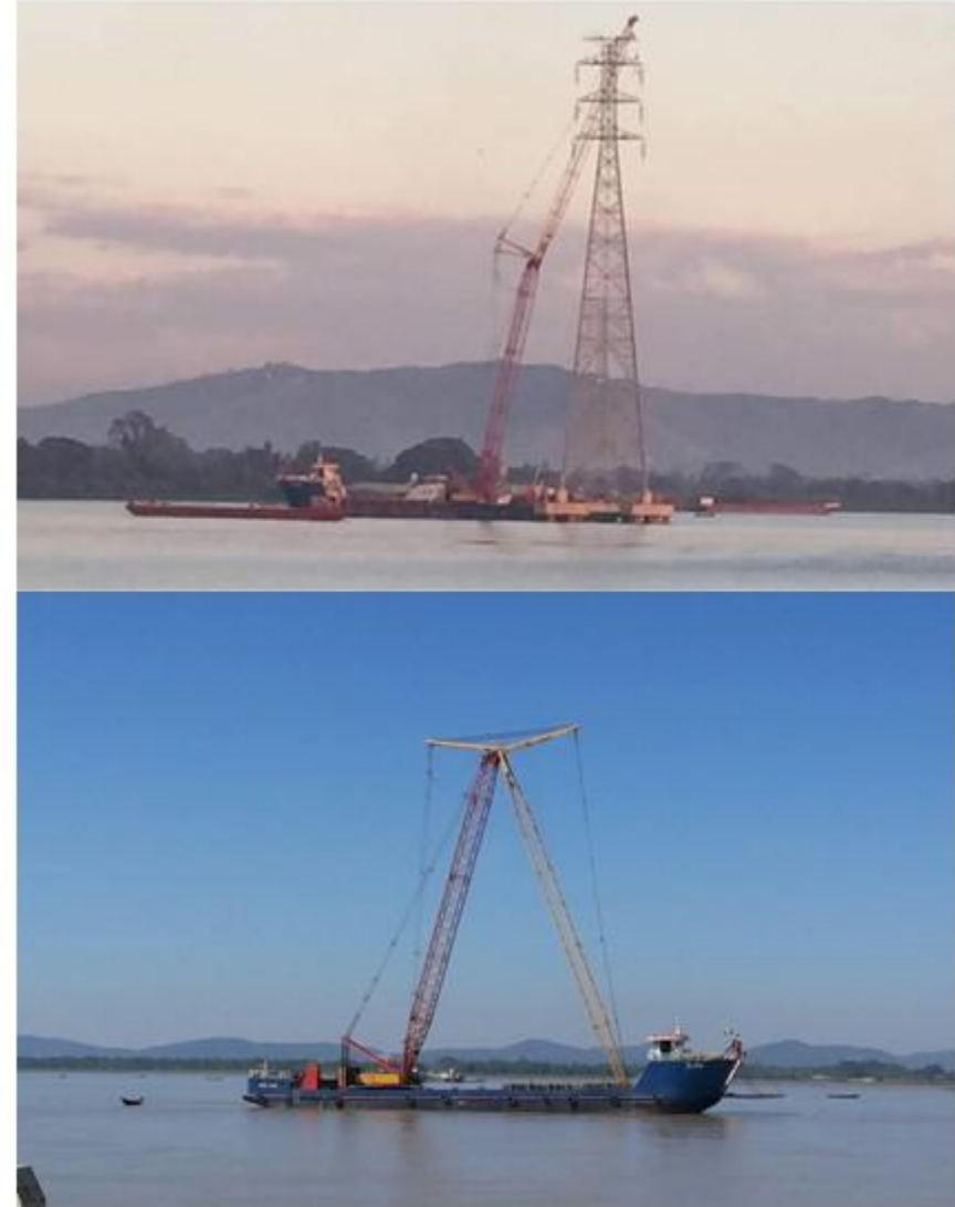
Tower Erection in Progress
