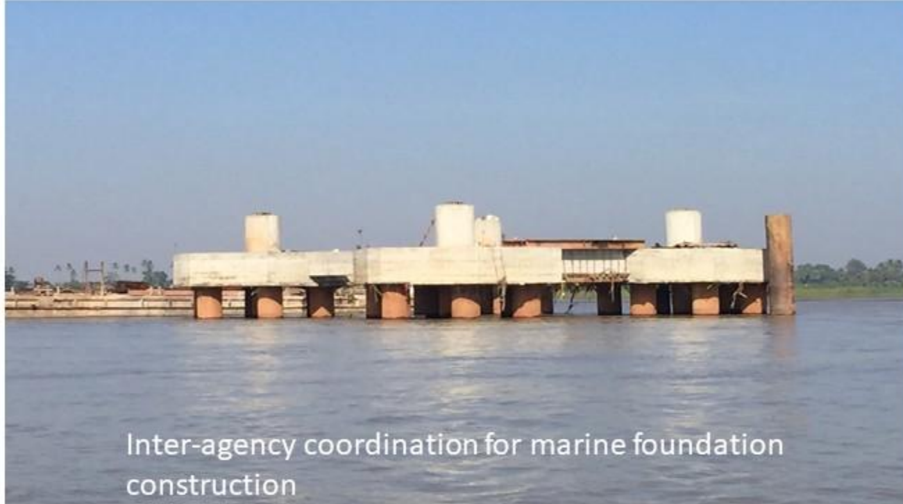
Foundation of River Crossing Tower
