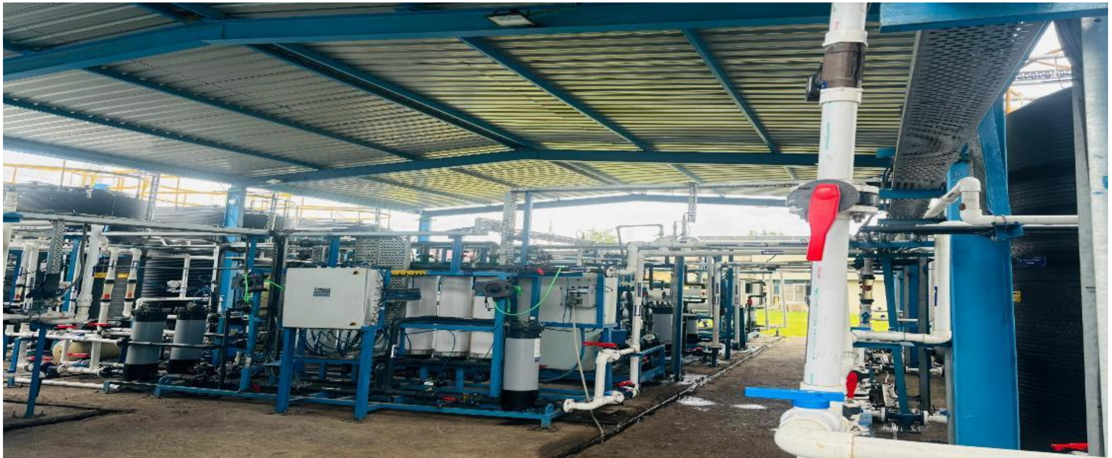
240 TPD Plant Non-Thermal Forward Osmosis based Water Purification Plant at NTPC Mauda Suited for Water having Calcium, Magnesium Hardness Under Operation
