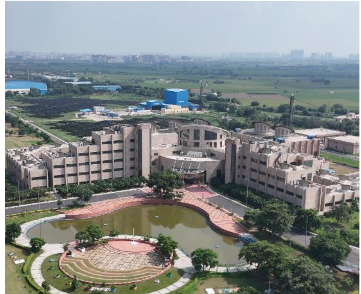
NETRA Main Building
